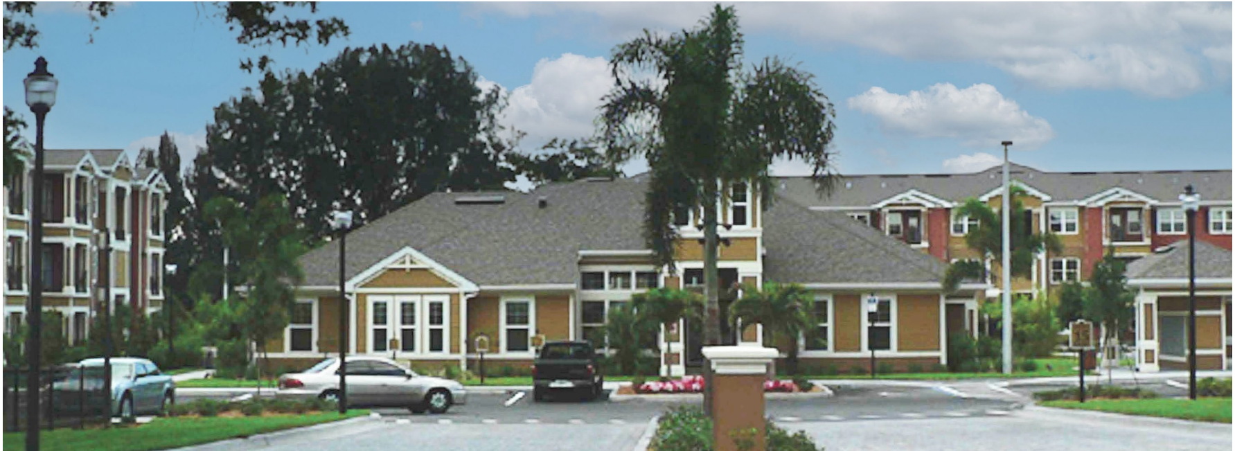
Developed by the Richman Group, Booker Creek in St. Petersburg offers 156 affordable rental units. It was constructed with financing from FHFC along with $850,362 of SHIP.
