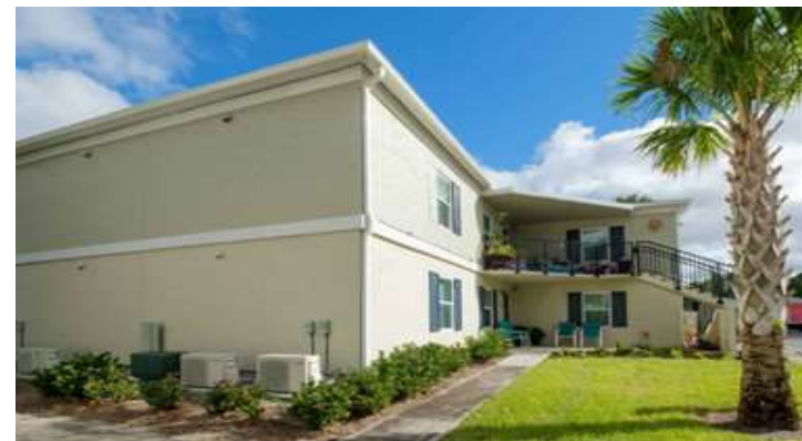
Wayne Densch Center Orlando, FL
