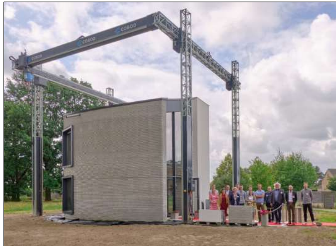
COBOD Printer doing a Two-Story House Print
