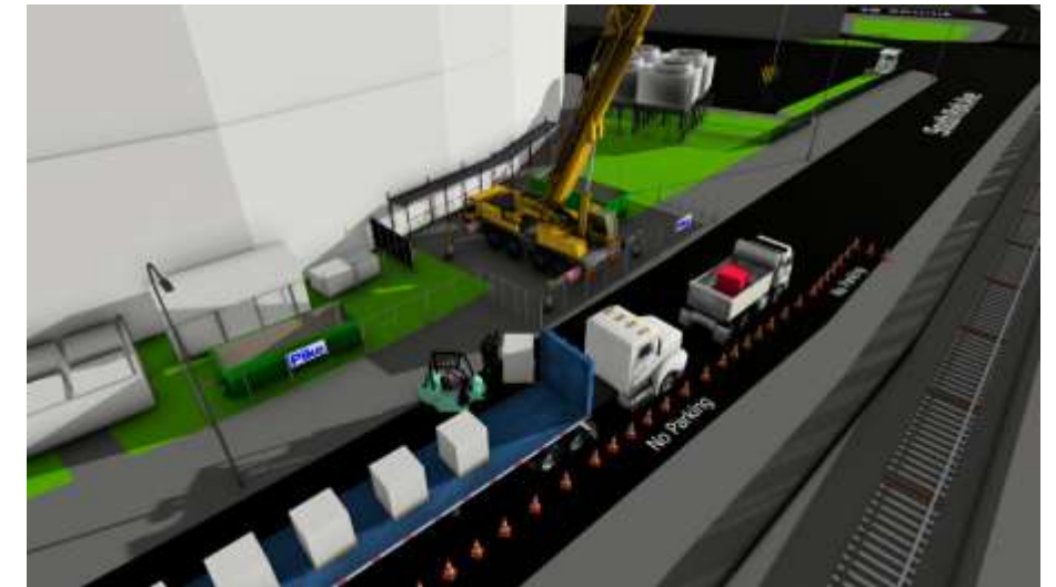
Material Delivery & Staging
