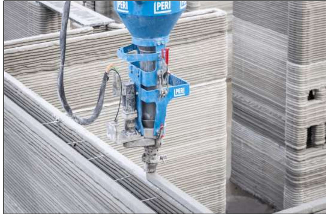
A Brief Introduction to 3D Printing of Concrete
