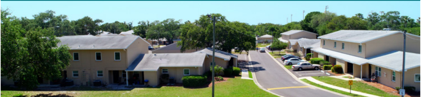
The Norton Apartments in Clearwater are owned and managed by the Pinellas County Housing Authority. SHIP has paid for rental rehabilitation in recent years.
