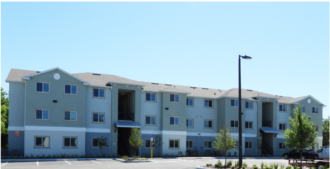
Tanager Square Apartments opened in 2024 in Pasco County, with 88 units which includes 15 SHIP units financed through SHIP funding. All units are fully leased. Tanager Square amenities include a cyber lounge, swimming pool, clubhouse, dog park, community room, and fitness center.
