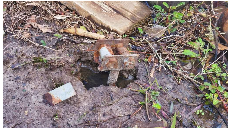
Anchor No Longer Attached
