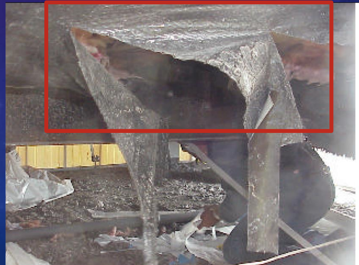
One of many penetrations in belly board
