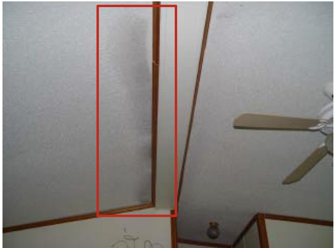
“Staining” of ceiling near marriage line
