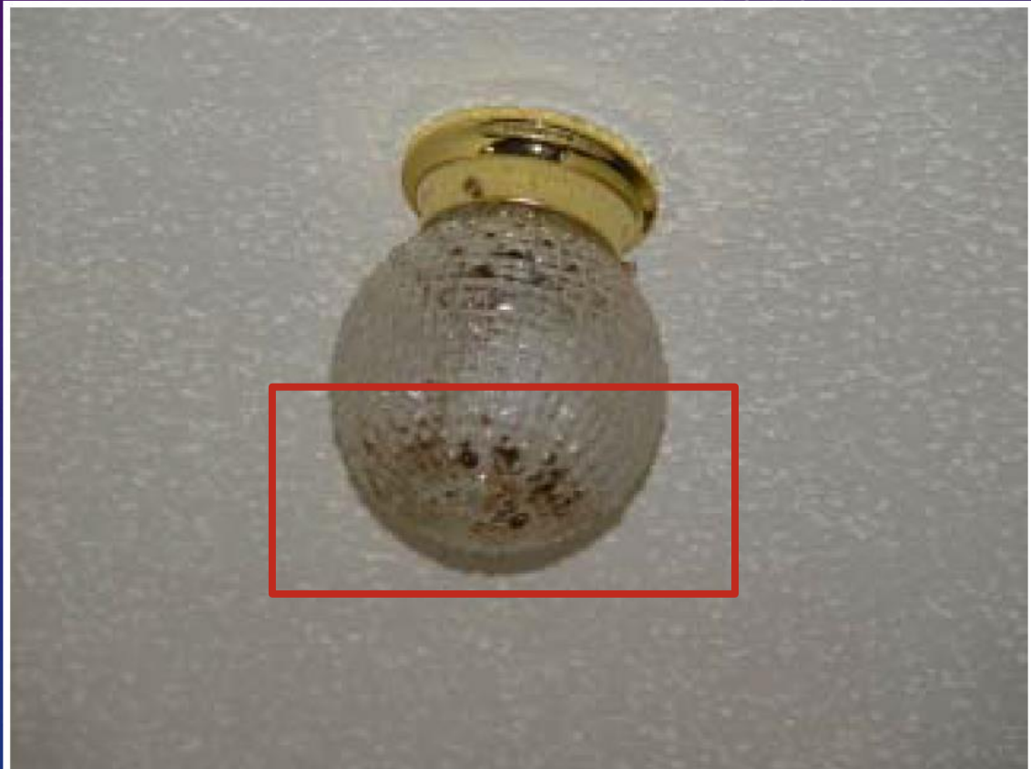
Hallway ceiling fixture with evidence of moisture within the globe
