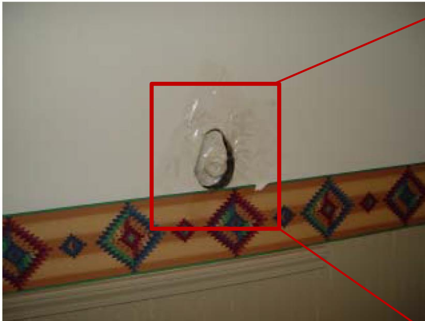
Master bedroom marriage line wall doorknob damage as a result of humidified materials
