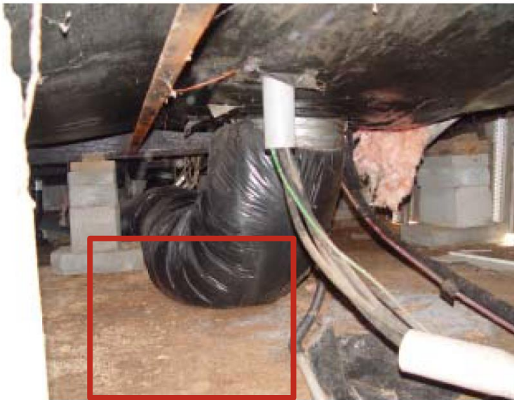
Crossover duct at air handler unit
