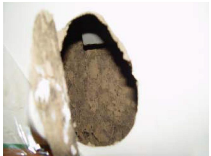
Evidence of biological growth within the marriage line wall assembly common to master suite and kitchen.
