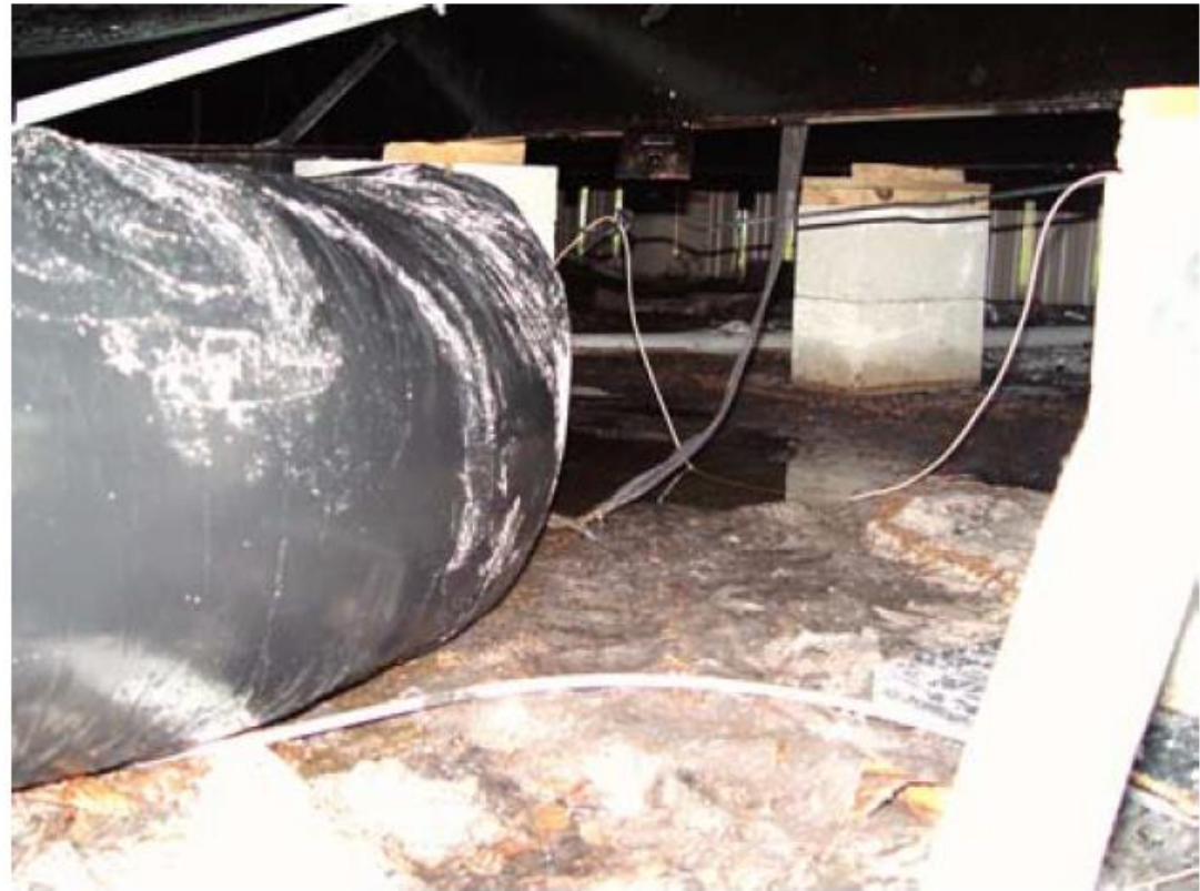
Figure 3. Standing water under house. Also note the duct work resting on the ground, absorbing the standing water.
