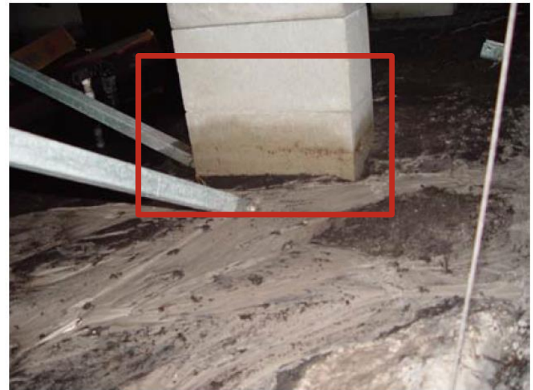
Figure 4. Flow lines under house, indicating running water under the house. Also note the “tide line” again.
