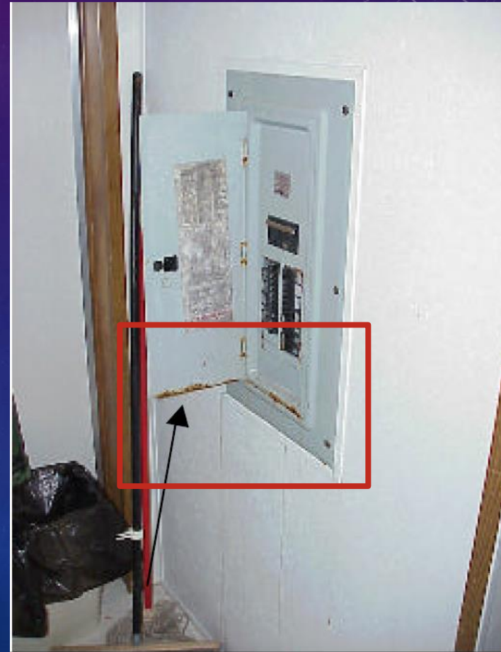
Rust on electrical service panel
