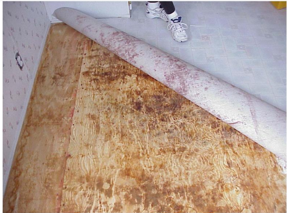
Figure 8 The floor covering has been partial removed. The plywood flooring was wet to the touch and staining exists on much of the under side of the vinyl. The floor decking was removed to inspect the underside – it appeared dry.
