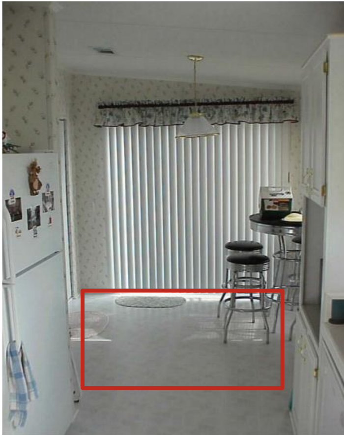
Figure 7 Breakfast nook with a vinyl floor covering and overhead supply register. Visible discoloration of the floor (pink spots) existed primarily in the area between the table and the cabinets on the right side of the picture. The supply register was oriented as to blow air to the outside wall.
