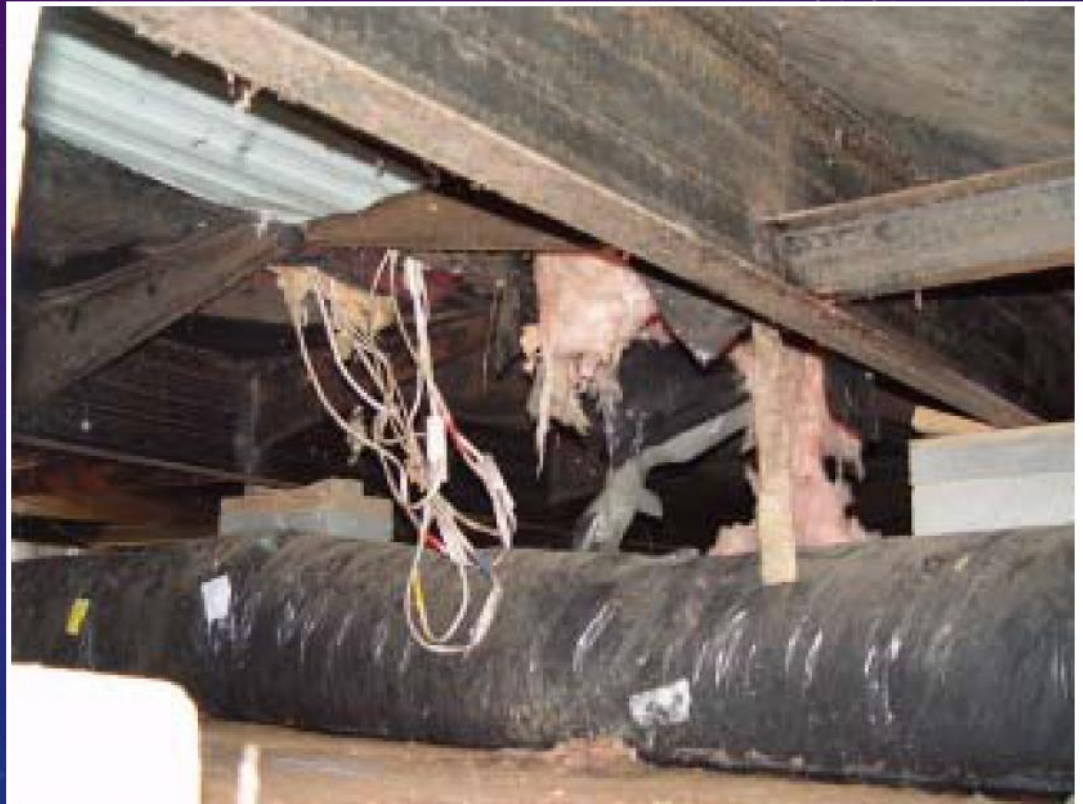
Compromised belly board at marriage line
