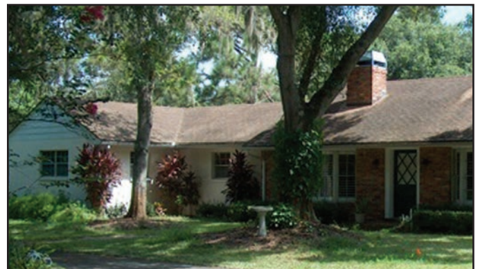
A small assisted living facility in Tampa.
