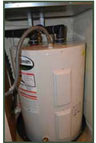
New energy efficient water heaters were installed.
