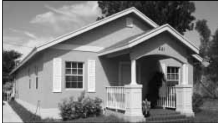
621 32nd Street: recently completed Northwood Renaissance CLT home in West Palm Beach.
