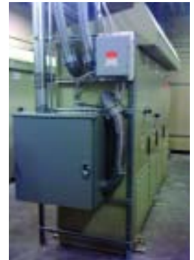
Inverters convert DC solar power to synchronized power
