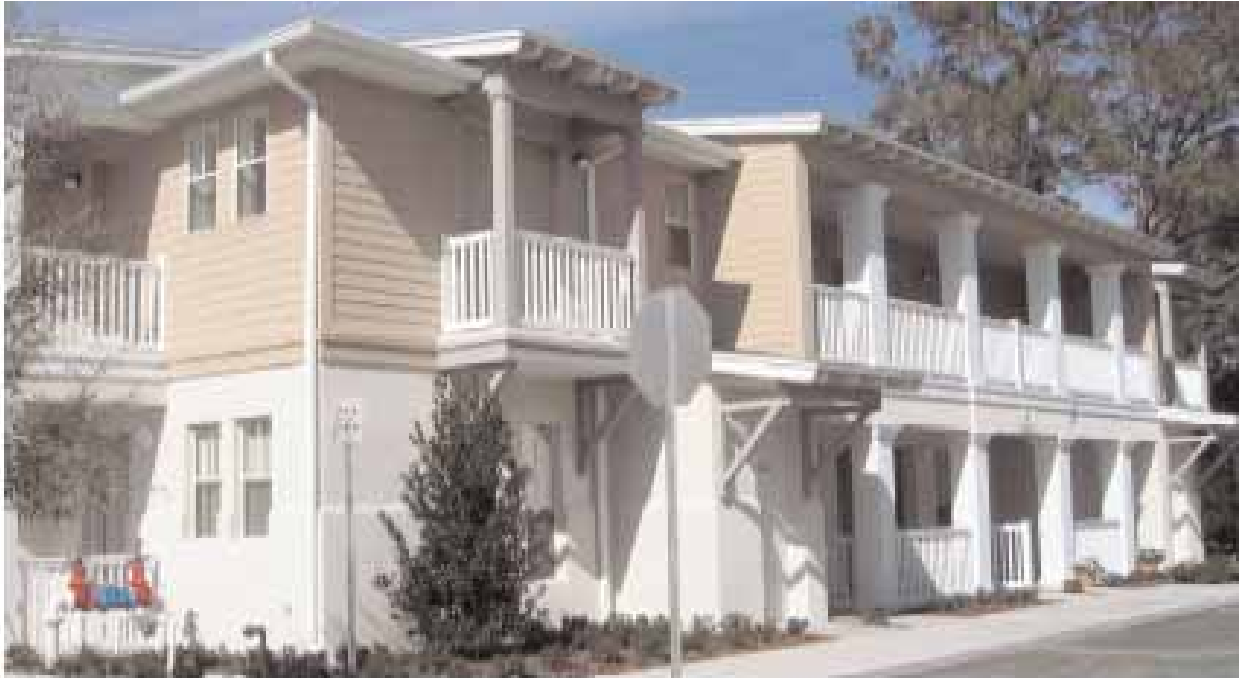
Railroad Avenue Apartments: The City of Winter Park provided over one million dollars from a combination of local government funds generated from a linkage fee ordinance and other local government initiatives to leverage Federal HOME funds and provide 30 units of new construction rental for low income families developed by Orlando Neighborhood Improvement Corporation. Partners included the Winter Park Housing Authority (which is leasing the land from the city) the nonprofit developer, Orlando Neighborhood Development Corporation, the Orange County Housing Finance Authority, Florida Community Partners, and Florida Community Capital Corporation. 12 units house very low income families; 10 units house low income families; and 8 units are market rate, no income restrictions.
