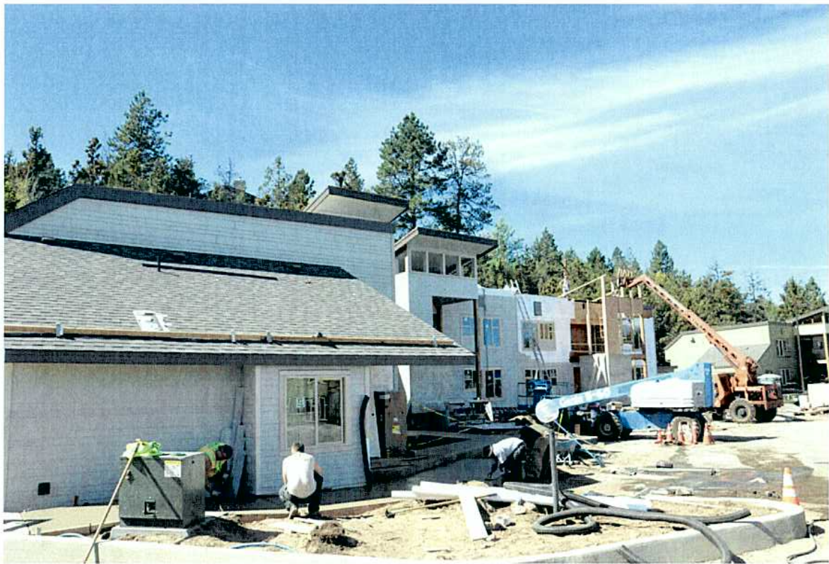
Figure 5 Construction at Crest Butte Apartments - Bend, OR
