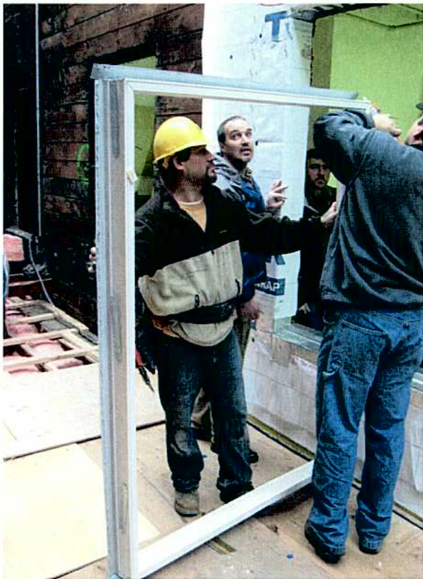
Figure 6 Window installation at Musolf Manor - Portland, OR
