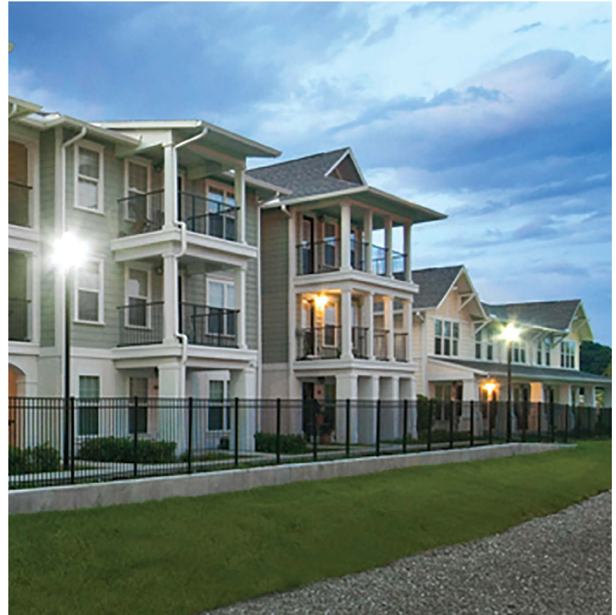
Located in Sarasota, Janie's Garden Phase I is an 86-unit complex comprising public and low income housing along with 20 market rate apartments.
