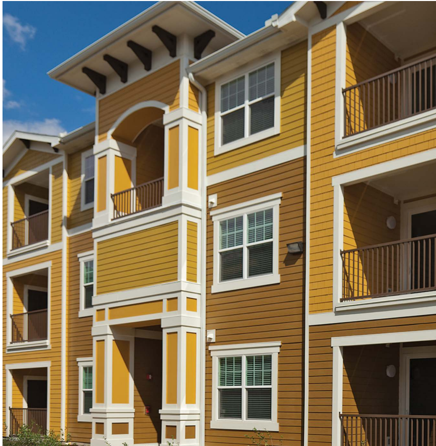
Bennett Creek is a 264-unit, multi-family housing community developed by the Richman Group to serve low income residents in Jacksonville. Its amenities include a pool, fitness center, laundry facility and grilling area.
